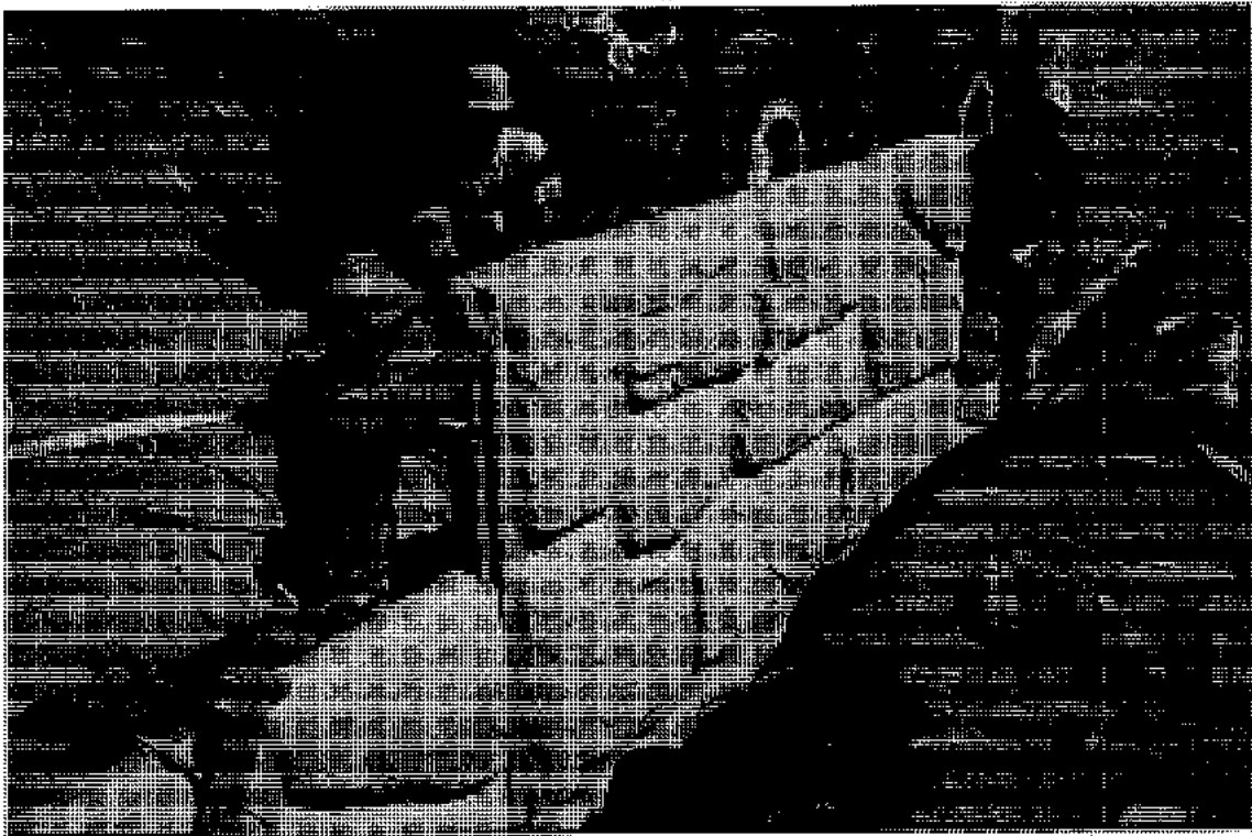
Placement of first lift of panels on leveling pad.
