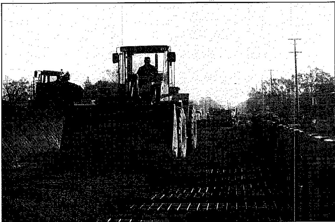
Spreading of backfill over installed reinforcing mesh.
