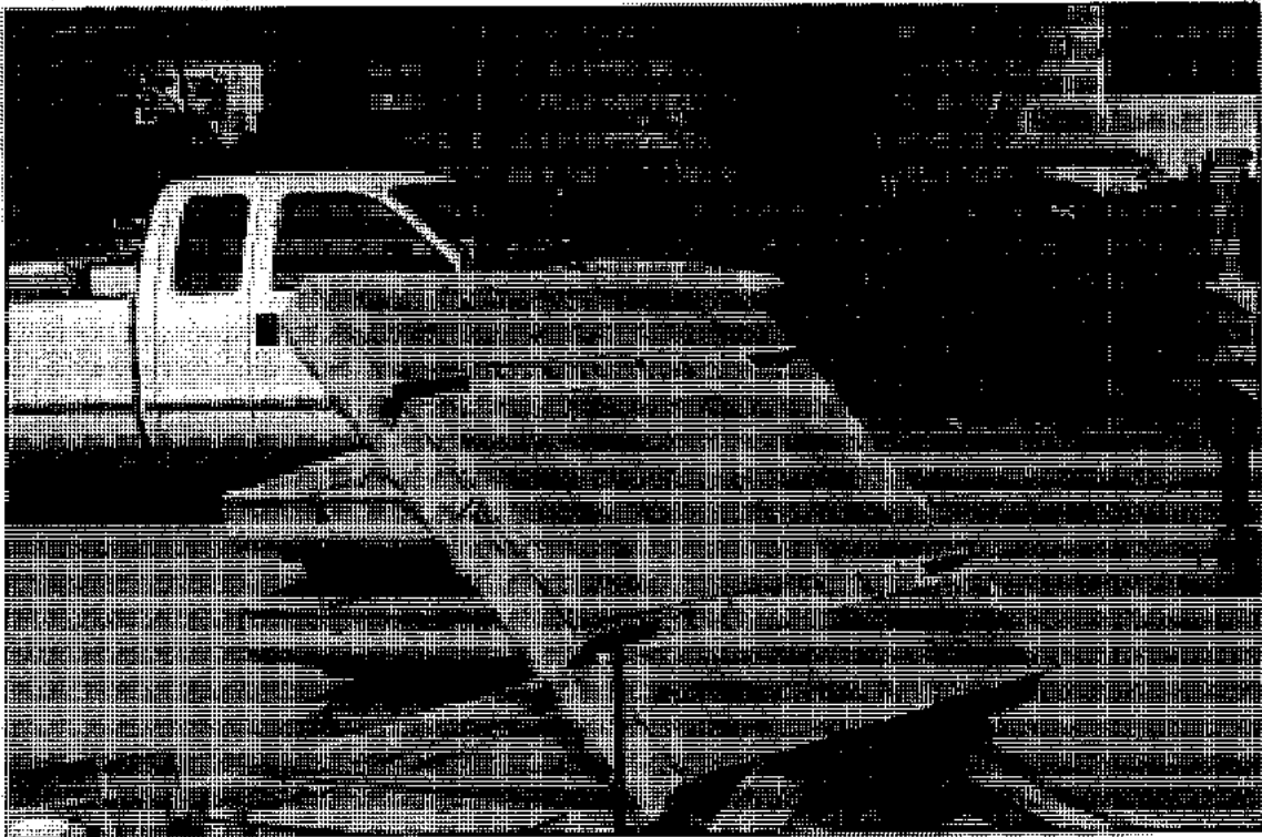
Hoisting of panel from stack with protective dunnage.
