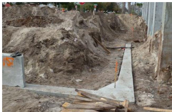
Figure 2-6. Leveling Pad at Corner
