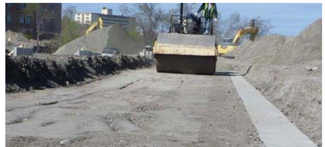
Figure 2-4. Foundation Preparation
