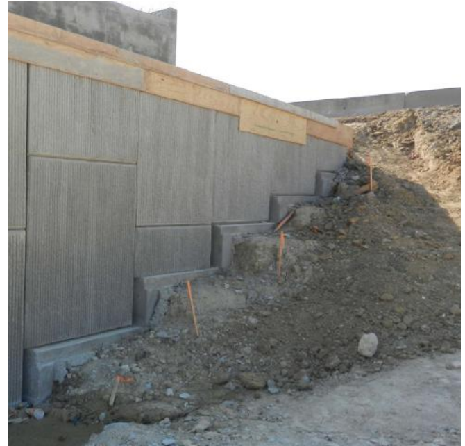
Figure 2-7. Leveling Pad Step
