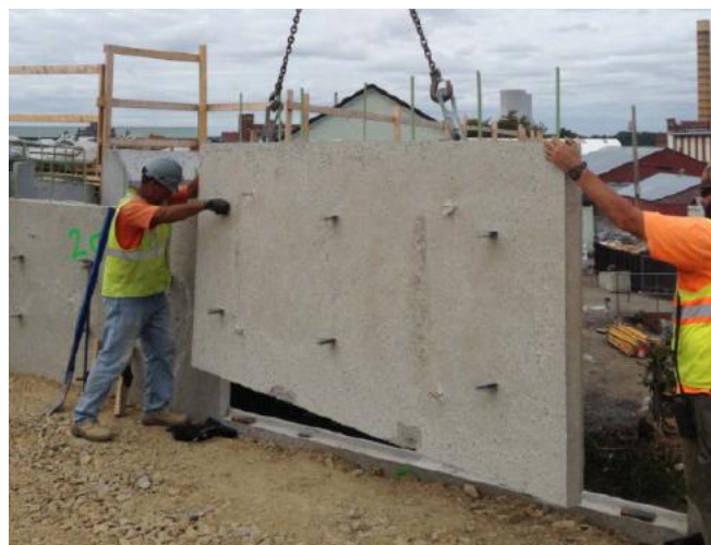
Figure 2-20. Setting Intermediate Panel
