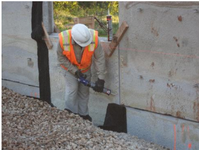
Figure 3-7. Filter Fabric Placement
