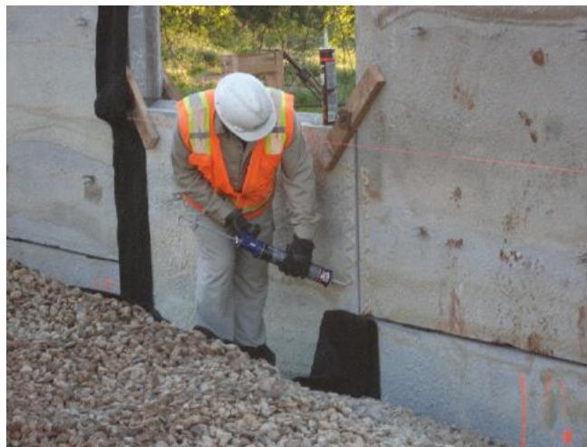
Figure 1-4 Application of Geotextile Adhesive
