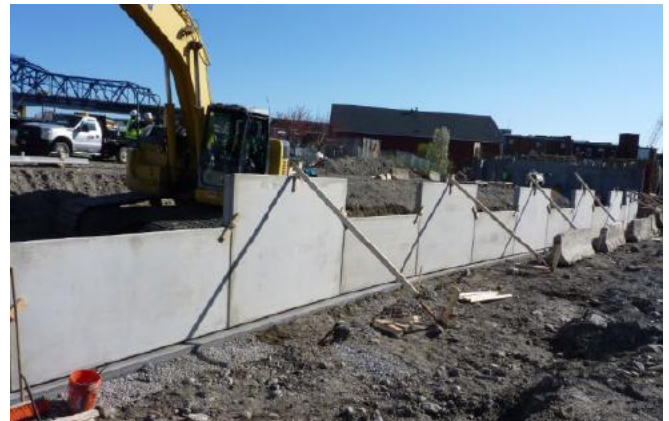
Figure 2-11. Bottom Panels Braced and Clamped
