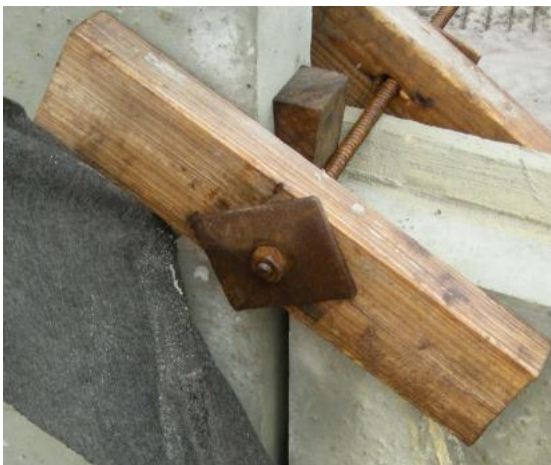
Figure 2-10. Typical Wood Panel Clamp
