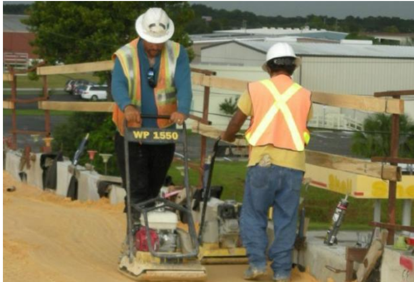
Photograph 3-1 Compaction of 3-Foot Zone
