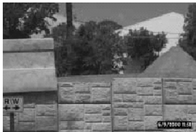
Figure 2-21. Mortar bedding on top of panels
