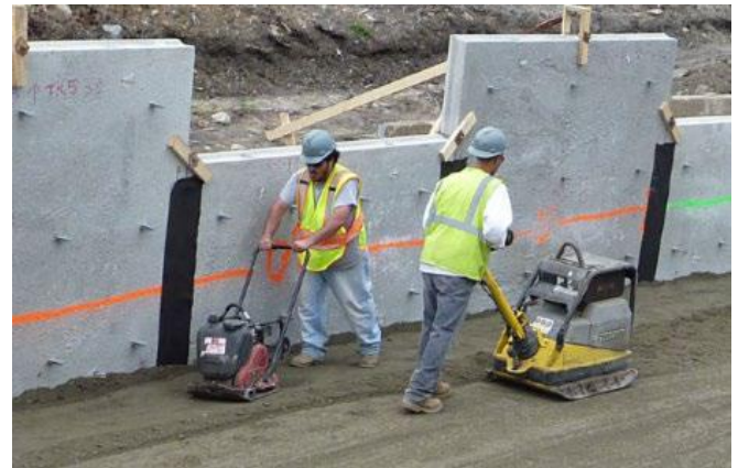
Figure 2-14. Hand Operated Equipment in 3-Foot Zone
