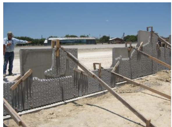
Figure 2-8. Bottom Panel Bracing
