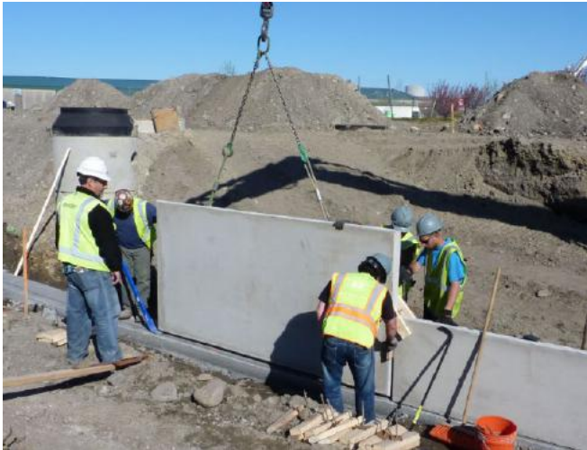
Figure 2-9. Setting and Clamping Panel
