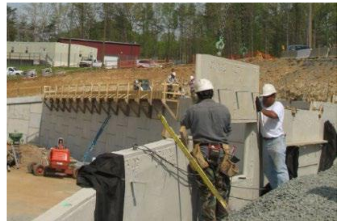
Figure 3-2. Facing Panel Lifting
