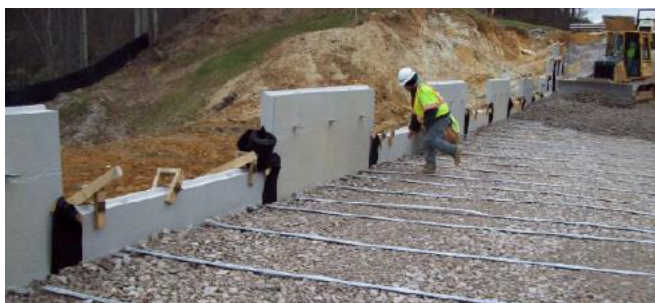
Figure 2-19. Spreading Fill on Compacted Lift
