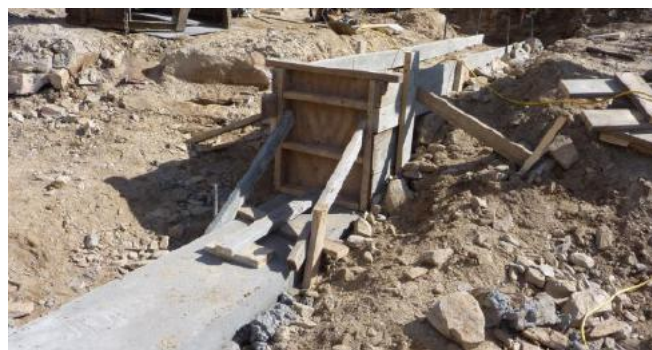
Figure 2-5. Leveling Pad at Step
