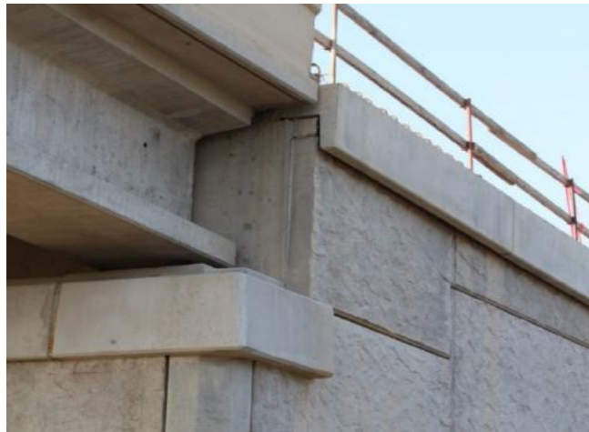
Photograph 1-1 Coping Unit at Top Facing Unit
