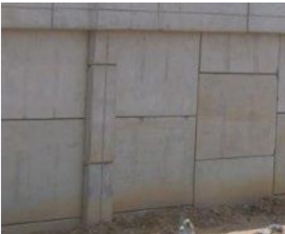
Figure 3-10. Slip Joint Detail
