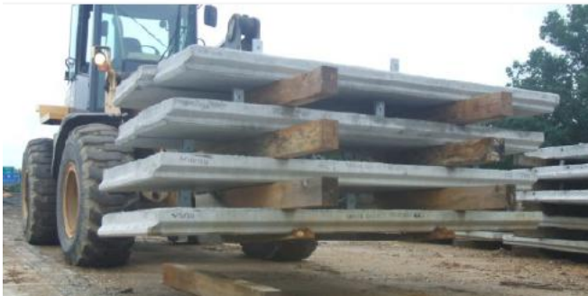
Figure 3-4. Panel Lifting with Dunnage
