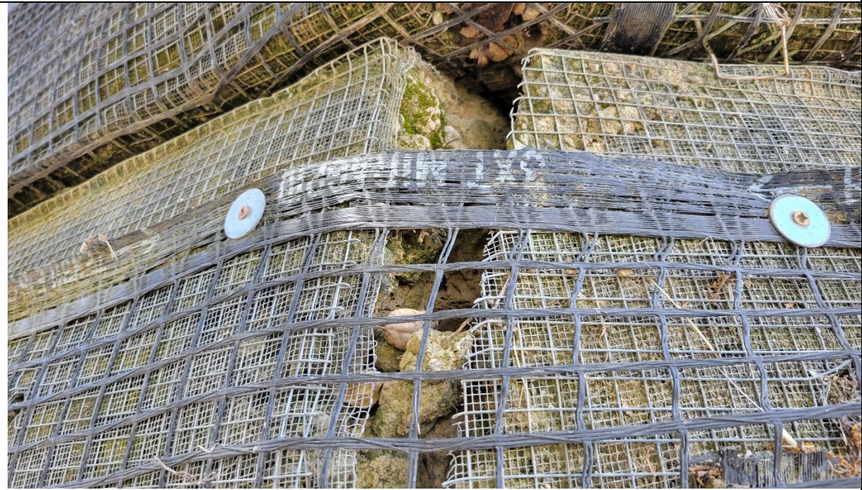
Photo 6. Cut corner units, geogrid anchored with screws and washers.
