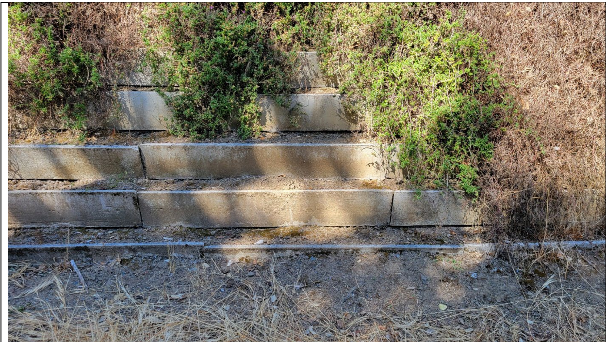
Photo 5. Toe of wall, where concrete planter panels exposed from vegetation.
