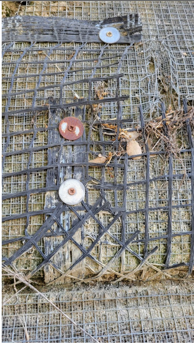
Photo 7. Anchor screws and washers, one corroded.
