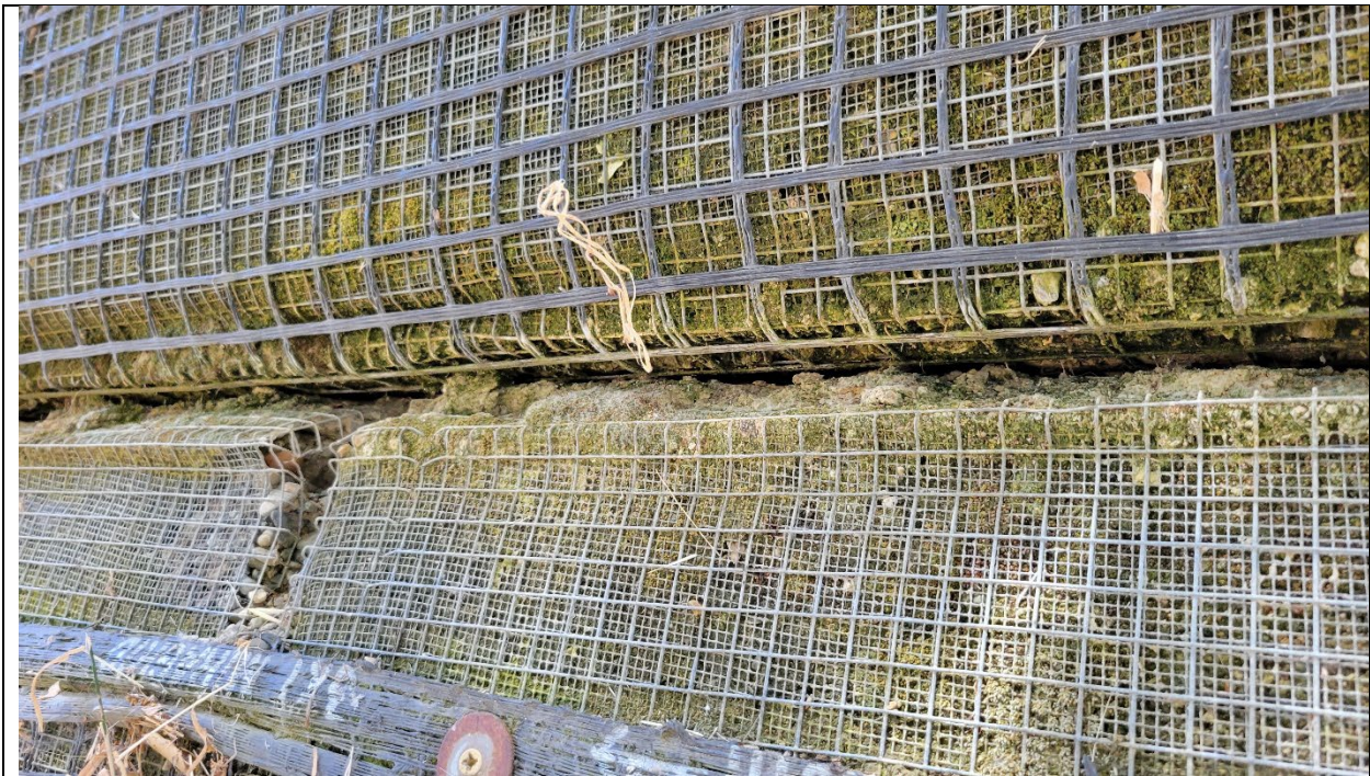
Photo 5. Face of wall close-up; face has metal screen and mesh, geogrid is wrapped up face of unit above.
