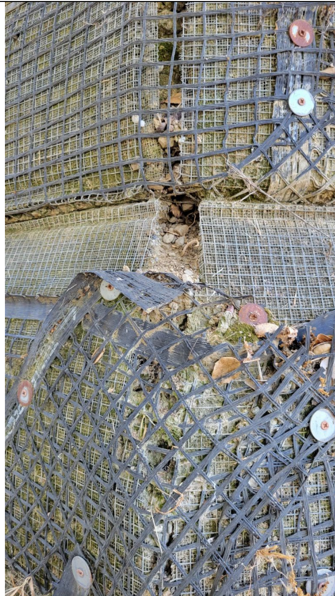
Photo 10. Geogrid anchorage at corner.
