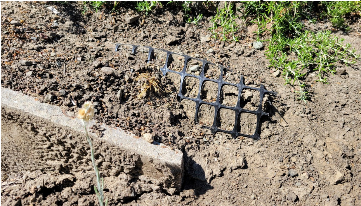
Photo 6. Top of wall, at a step down, where geogrid wrap on face is exposed.
