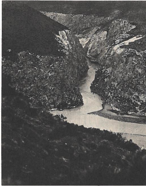
FIG. 3.—Aguada Blanca Canyon Seen from Upstream Prior to Damming; On Left Bank, Ignimbrite Appears Covered by Dark Piroclasts
