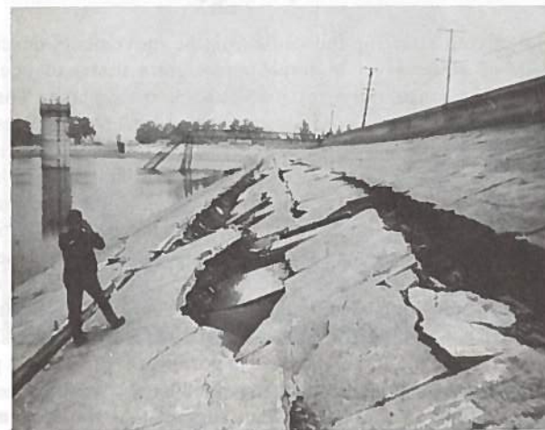
FIG. 8.—Slide Scarps on Upstream Face of Embankment
