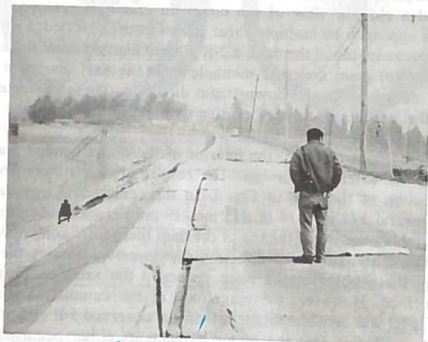
FIG. 7.—Deformation of Parapet Wall Resulting from Downstream Movement of Embankment
