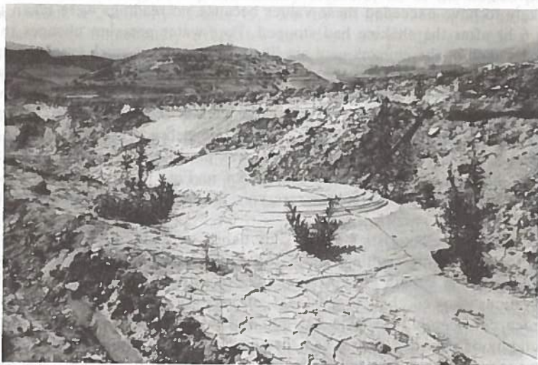
FIG. 12.—Sand Boils in Depression Scarps near Toe of Slide Debris, Lower San Fernando Dam
