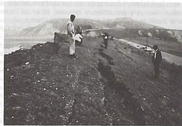
FIG. 10.—Longitudinal Cracks in Remaining Portion of Embankment, Lower San Fernando Dam
