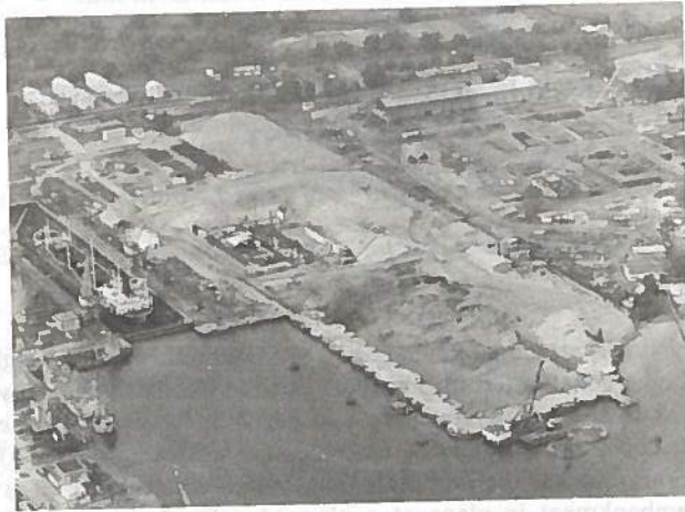
FIG. 1.—Sembawang Dry Dock Under Construction. (Western Embankment Is in Lower Right, where Two Sheet Pile Walls Are Visible)
