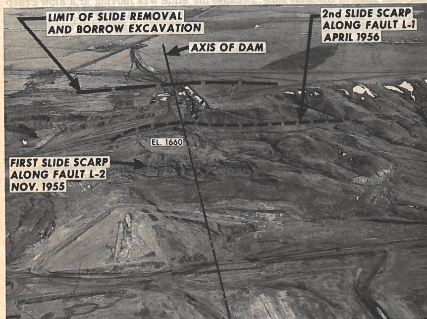
FIG. 6.—AERIAL VIEW OF SLIDE, LEFT ABUTMENT, MARCH 20, 1956
