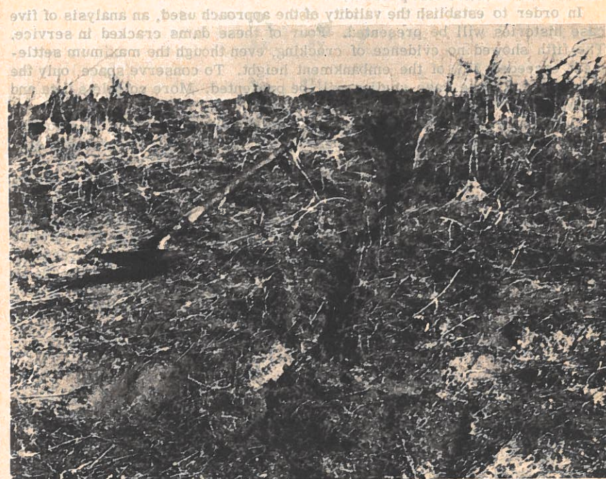
FIG. 2.—WOODCREST DAM: CLOSE-UP OF TRANSVERSE CRACK (JANUARY, 1960)
