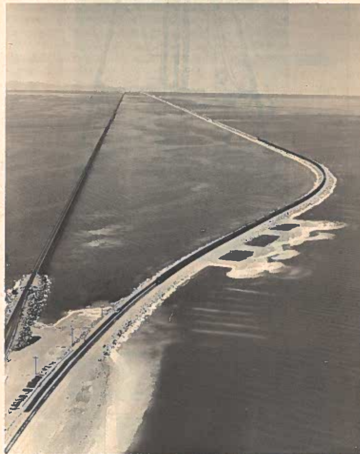
FIG. 7.—AERIAL VIEW OF GREAT SALT LAKE RAILROAD FILL, LOOKING WEST
