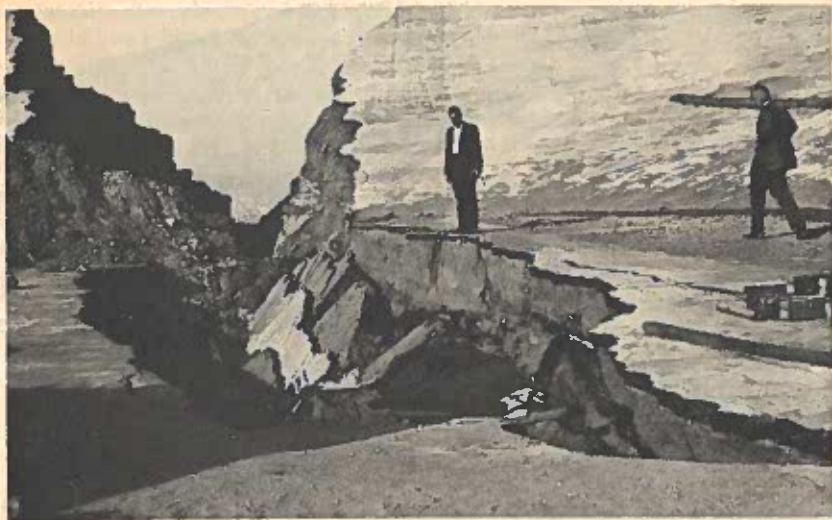
FIG. 20.—LARGEST SINK HOLE ALONG FAULT MERGED WITH CREVASSE
