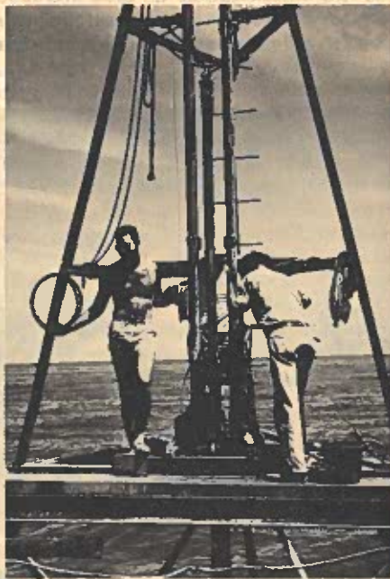
FIG. 8.—SWEDISH FOIL SAMPLER OPERATING IN GREAT SALT LAKE FROM A PORTABLE TRIPOD
