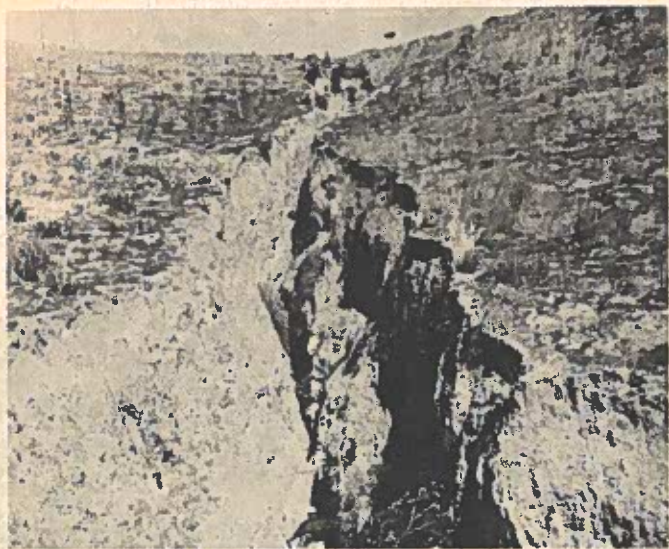
FIG. 21.—ILLUSTRATION OF ERODIBILITY OF INGLEWOOD FORMATION IN WHICH THE BALDWIN RESERVOIR WAS CONSTRUCTED (GULLY IS ABOUT 40 FT DEEP)
