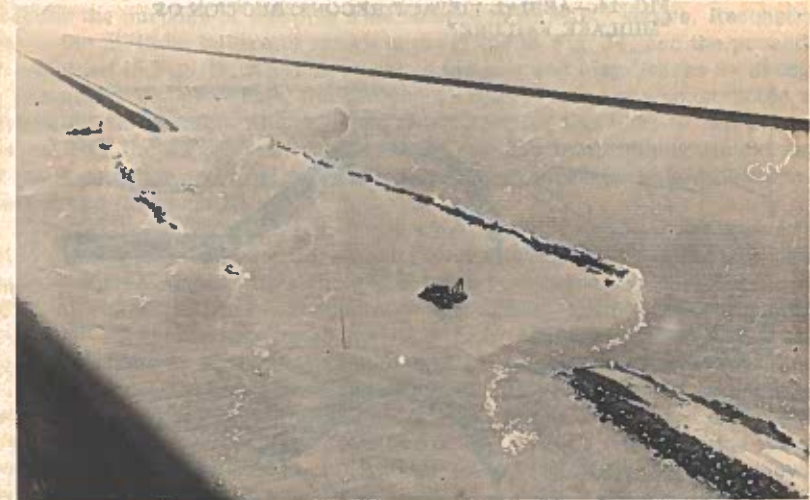
FIG. 13.—AERIAL VIEW OF "MIDLAKE FAILURE"
