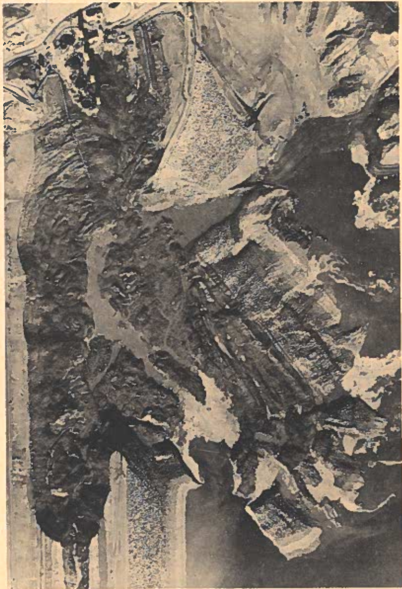
FIG. 2.—AERIAL VIEW OF SLIDE IN FORT PECK DAM
