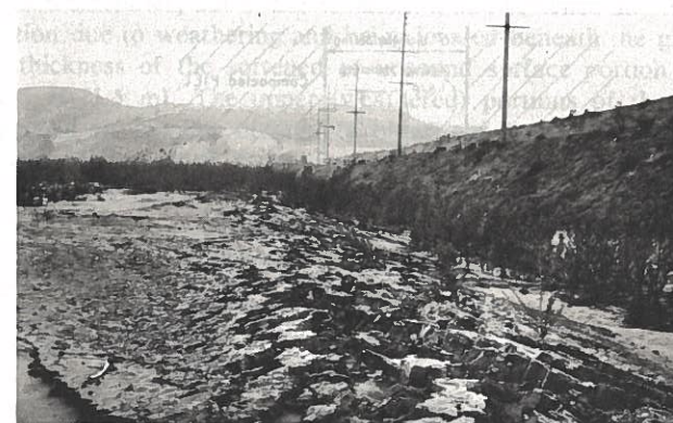
FIG. 8.—Pressure Ridge (Looking South Along Toe of Fill Slope)
