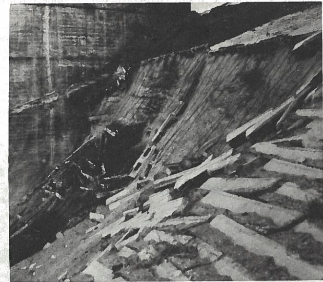
FIG. 6.—Liqufaction Failure on South Side of Morning Glory Spillway—Kingsley Dam
