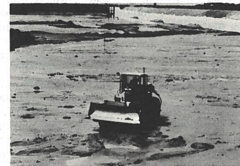
FIG. 12.—Compactive Hydraulic Fill with Rubber-Tired Rollers—Greenville Fill—Mississippi Power and Light Power Plant
