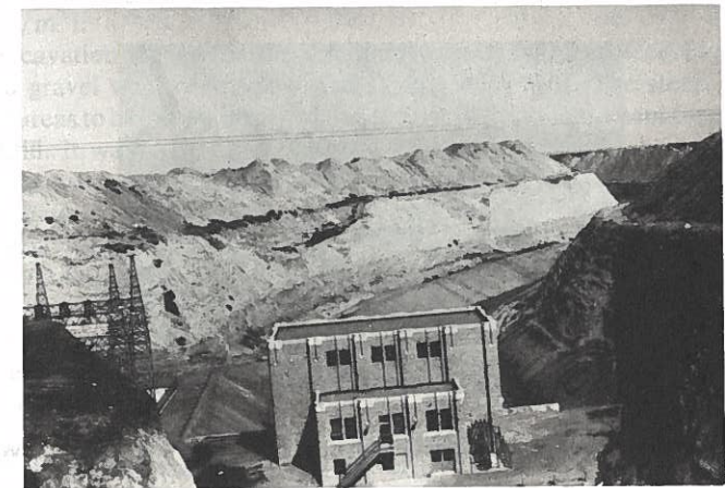
FIG. 7.—Johnson No. 2 Powerhouse with Backfill in Place (Note Steep Slopes)
