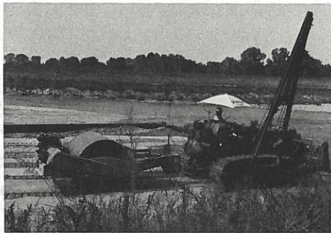
FIG. 9.—Vibrating Roller for Compacting Hydraulic Fill for Rush Island Power Plant
