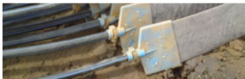
Connecting PVD to fitting cap
